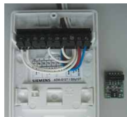
Typical simple E-Line wiring
