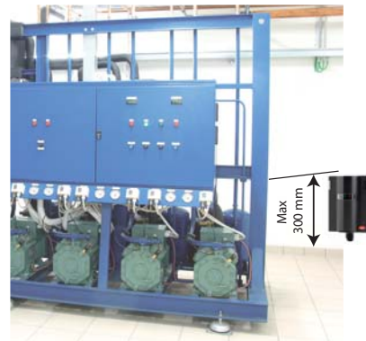
For gas: R22 - R134a - R404a - R407a, R407c - R407f R410A - R507a - R290 - CO2 h max 300 mm
